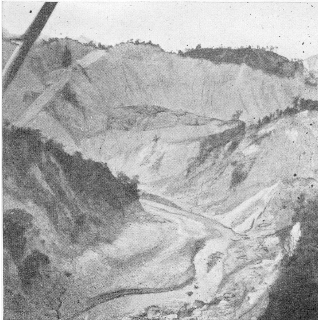
Example of slope failure in Assam earthquake of 15 August 1950 in India. The figure shows the damaged valley of the river Simen north of Dibrugarh [After Gee (1953)]
